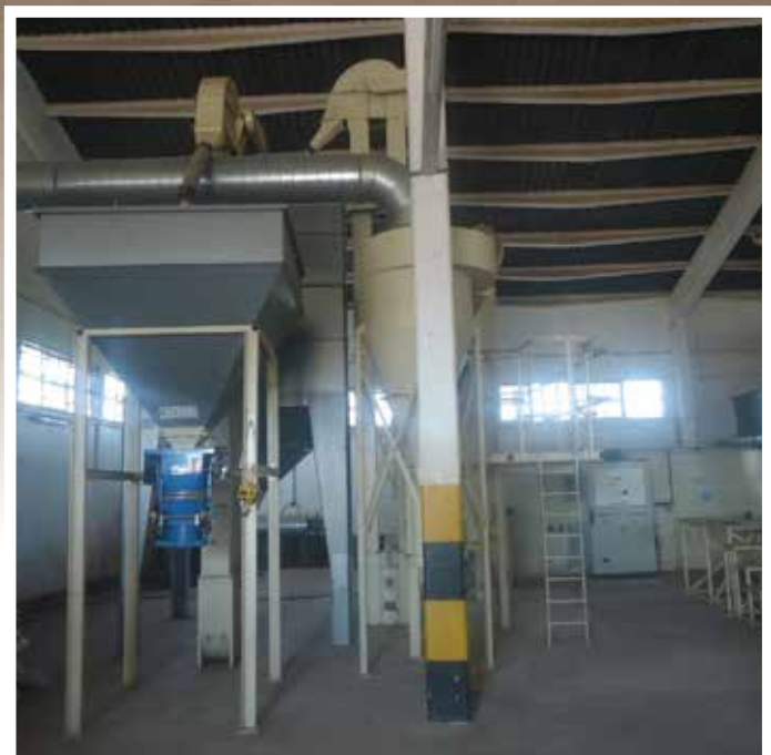
The Gulu storage warehouse and facilities
